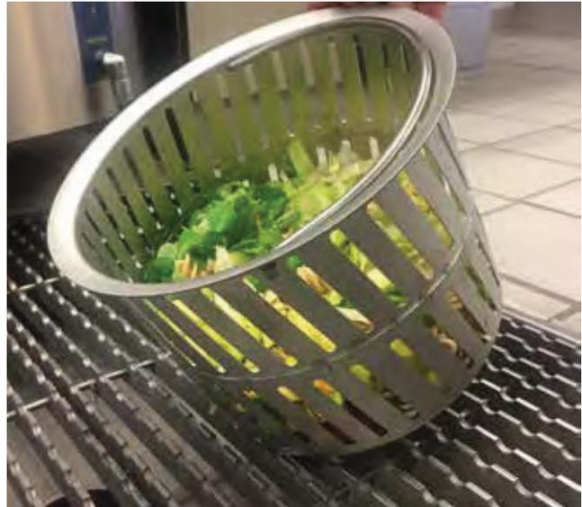
Figure 5. A 7-litre filter basket that is filled halfway allows full flow. A channel filter can hold back waste before it enters the channel.
